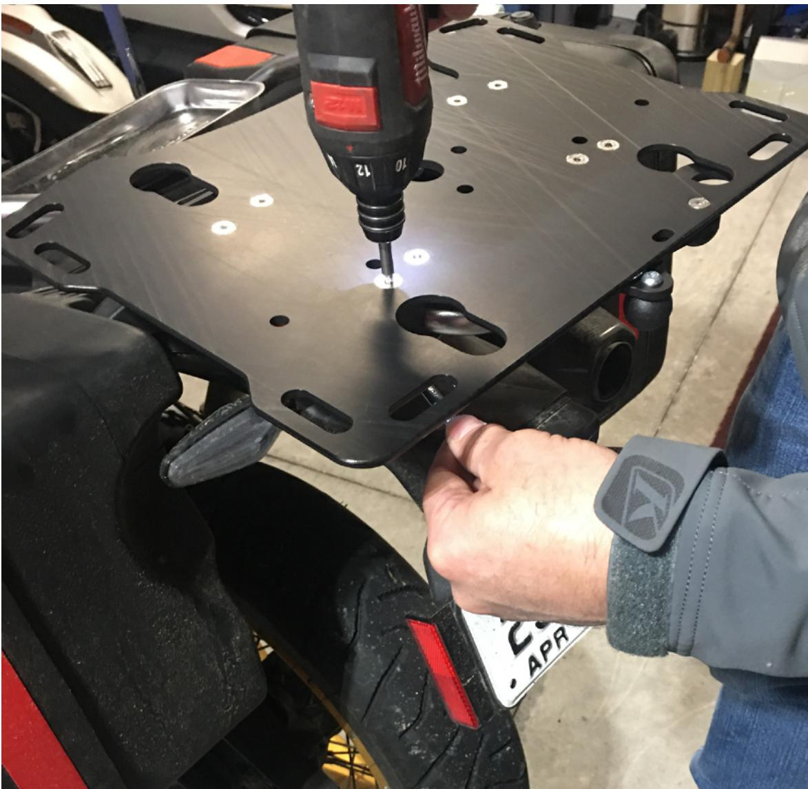
**Step 6** Use a 4mm driver and 10mm open end wrench to tighten all eight M6 lock nuts. **Note:** Clamp halves will be closed together when tightened correctly, do not over tighten.
