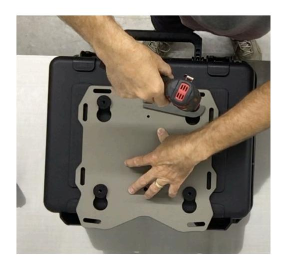
Step 10 With one hand apply downward force on the Slider plate, use your other hand to drill the case. With a 1/4" drill bit and electric drill use the master puck as a drill guide and drill a pilot hole through the box.
