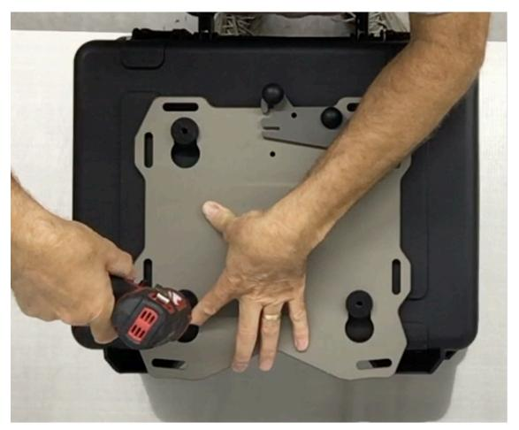
**Step 14** With the ¼" drill bit, use the puck diagonally across from the master puck as a drill guide and drill a second pilot hole in the case.
