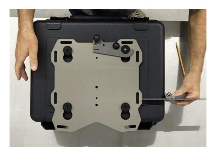
**Step 8** Place the Slider plate with the other 3 pucks onto the master puck and latch it into position. Square up the plate and box to each other (last chance). **Note: Apache 3800 case** verify the case ribs are seated in the puck grooves.
