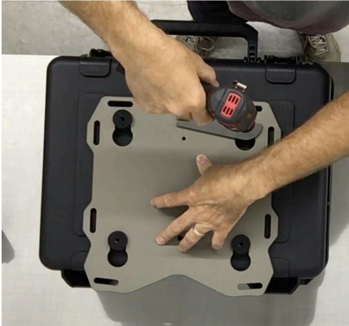
**Step 12** With one hand apply downward force on the Slider plate, use your other hand to drill the case. With a ¼” drill bit and electric drill use the master puck as a drill guide and drill a pilot hole through the box.
