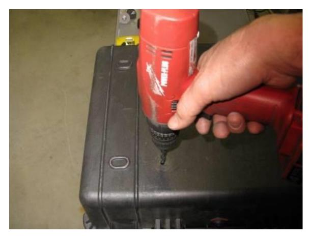
**Step 14** Remove the rack from the box. Use the 21/64" drill bit and electric drill to enlarge the ¼" pilot hole.
