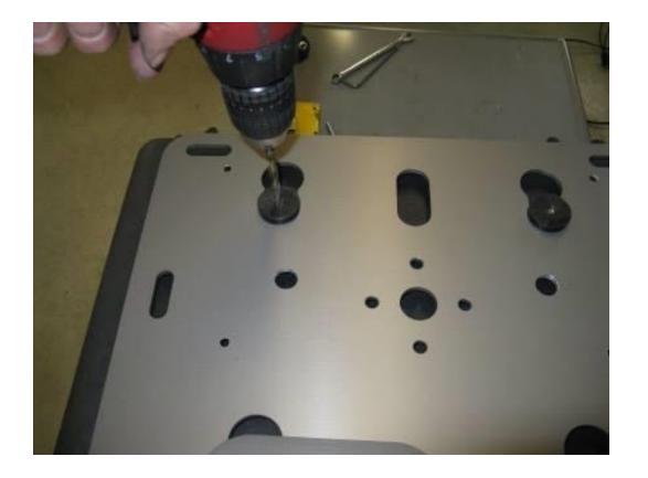
Step 20 Bolt the second puck to the box. Place the rack on the box and latch it into position. With the 1/4" drill bit use the 2 remaining pucks as drill guides and drill the last 2 pilot holes.
