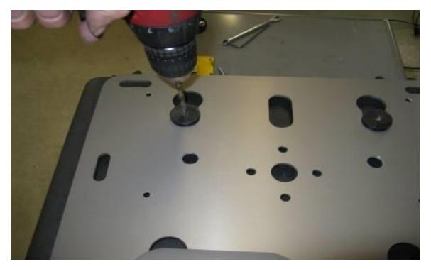
**Step 25** Bolt the second puck to the box. Place the plate on the box and latch it into position. With the 1/4" drill bit use the 2 remaining pucks as drill guides and drill the last 2 pilot holes.
