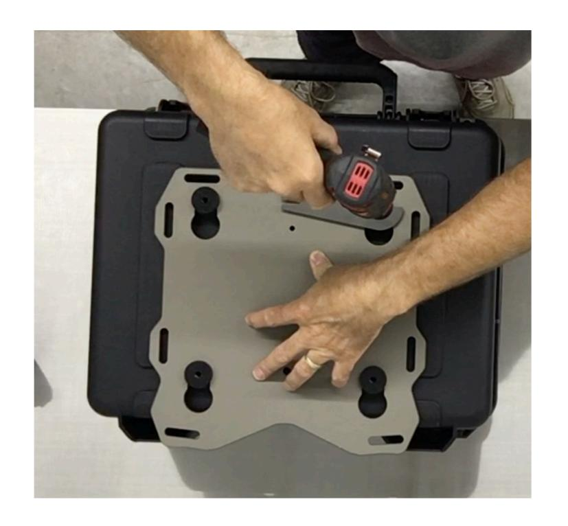
**Step 14** With one hand apply downward force on the Slider plate, use your other hand to drill the case. With a  $\frac{1}{4}$ " drill bit and electric drill use the master puck as a drill guide and drill a pilot hole through the case.
