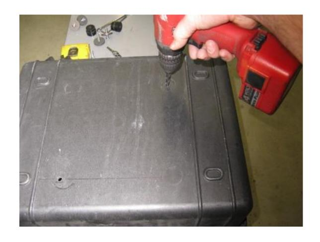
**Step 17** Remove the rack and pucks from the box. Use the 21/64" drill bit and electric drill to enlarge the second ¼" pilot hole.
