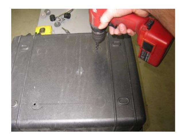
Step 15 Remove the plate and pucks from the case. Use the 21/64" drill bit and electric drill to enlarge the second ¼" pilot hole.
