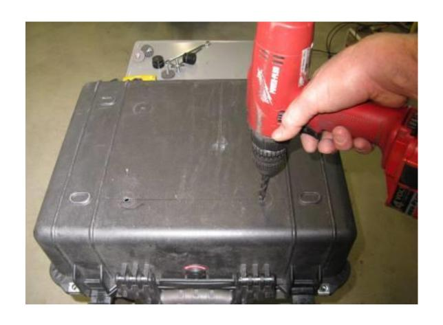
Step 13 Remove the rack and pucks from the box. Use the 21/64" drill bit and electric drill to enlarge the last 2 1/4" pilot holes.
